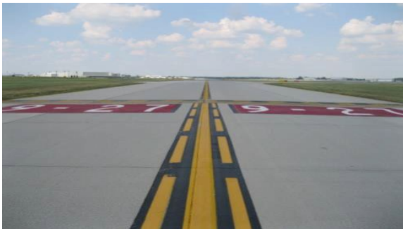
Enhanced Taxiway Centerline Marking
